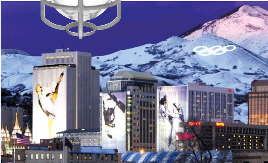
1,850 RAB Vaporproof Lights formed the Olympic Rings in the mountains above Salt Lake City
