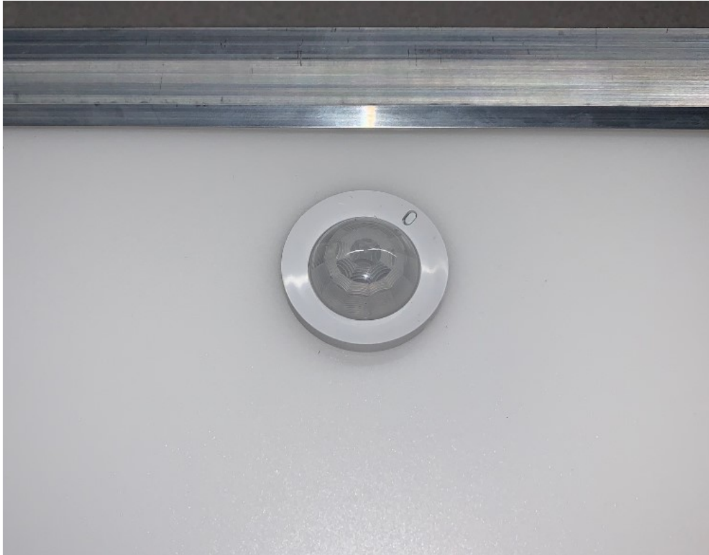
Figure 17: RES7 sensor optic snapped in place
