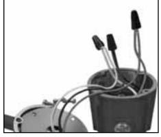
Make all necessary connections observing polarity, i.e. green-toground, white-to-common, and black-to-voltage.
