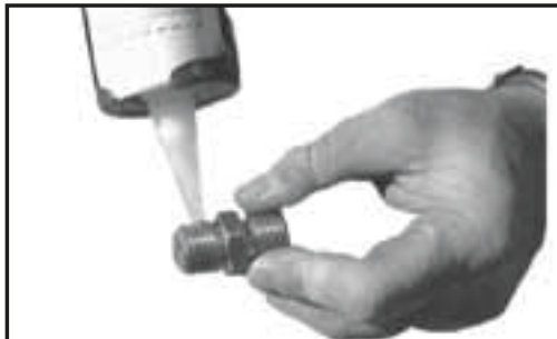
Step 1 - Coat coupling threads with thread sealant to keep moisture from entering junction box.
