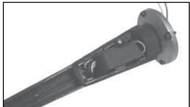
Step 5 - Remove half fixture. Remove transformer and replace with new transformer. Reassemble fixture in opposite order.
