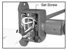
6. Adjust fixture and secure with set screw.
