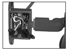
Make wire connections observing polarity, i.e., green-toground, white-to-common and black-to-voltage.
