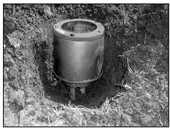
1. Excavate hole in desired location approximately 12" in diameter and about 3" deeper than height of fixture. Connect housing to conduit system using a good thread sealant.
