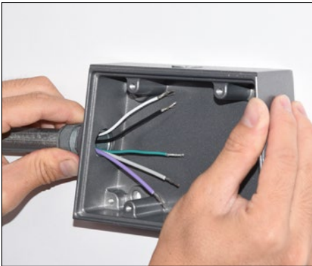
1. Install Conduit Line to Conduit Box. Note: Apply Thread Sealer to Conduit Nipple for a water tight seal.
