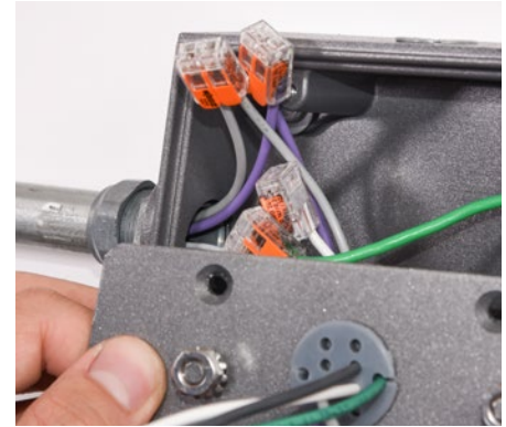
9. Hook up wire harness to the incoming line per the local electrical code.
