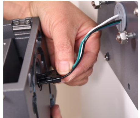
12. Run quick disconnect thru wire way on the back of the fixture.
