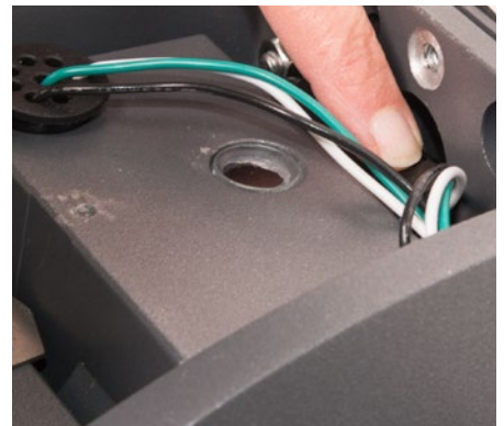
15. Tuck quick disconnect connector into back of fixture housing.
