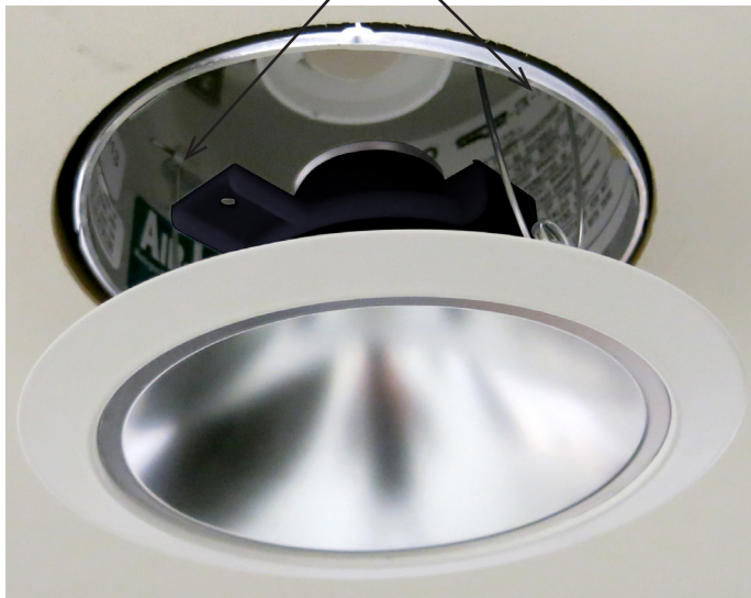
Figure 3 Install Springs
