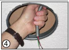
Step **9**: **Wiring:** Remove junction box cover and the appropriate knock-out(s) and connect conduit to junction box with proper connector (not supplied). Connect black fixture wire to hot, white fixture wire to neutral and green wire to ground (make sure all connections are tight). Place all wiring and connectors back in junction box and replace cover.
