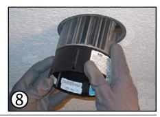
Step **9**: Align slotted holes (3) of housing with screw holes on housing ring and secure with 3 screws (supplied). Align edge of housing flush with ceiling before tighten screws. Make sure screws are fully engaged.
