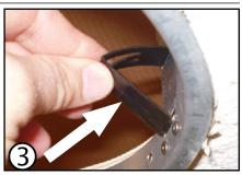
Step **4**: Pull power supply thru opening. Electrical service must meet your local electrical code and supply wire insulation must be rated for at least 90° C.
