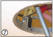
Step **3**: Push LED housing thru housing ring.
