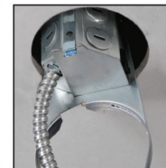
Insert plaster frame into ceiling opening.
