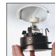
Insert trim to complete installation.
