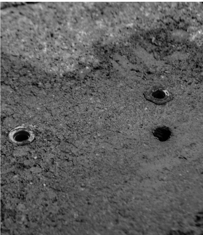
3. Insert anchor bolts into the two mounting holes Note: Do not use anchor bolt in the wire through hole
