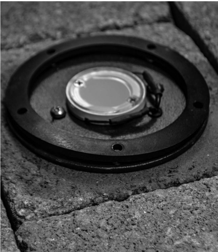
7. Place the gasket on the mounting plate
