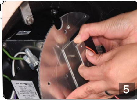
Pull existing driver tray from fixture.
