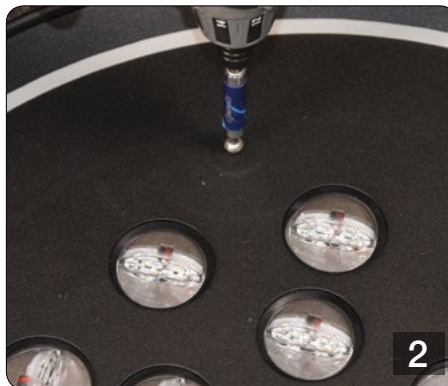
Remove (4) existing screws as shown. Discard screws. Pull out existing LED deck.
