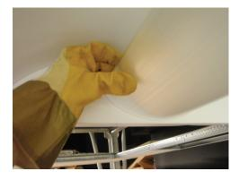
Allow opposite edge of basket to hinge on light seal during lamping and fixture maintenance. To replace baskets, refasten both ends of the shielding over the light seal.
