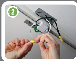
Connect track to mounting plate and wire.
