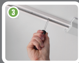
Attach track to ceiling.
