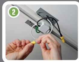
2 Connect track to mounting plate and wire.
