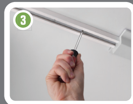
3 Attach track to ceiling.
