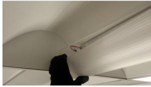
To remove the basket, grip the basket towards the end of the fixture. Rotate and Unhook the basket from the light traps. Store basket in a safe location where it will get damaged. Reverse the steps to reinstall.
