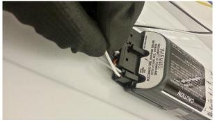
While supporting the reflector, plug in the test switch.
