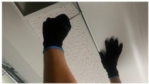
To gain access inside the channel, gently push upwards on the reflector with the test switch present until the notch in the reflector is visible. Insert a screwdriver into the notch to pry and wedge open.
