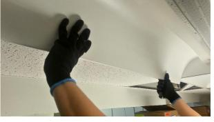
Once a corner of the reflector is freed from the channel, slide the screwdriver towards the other end of the housing to release the reflector.
